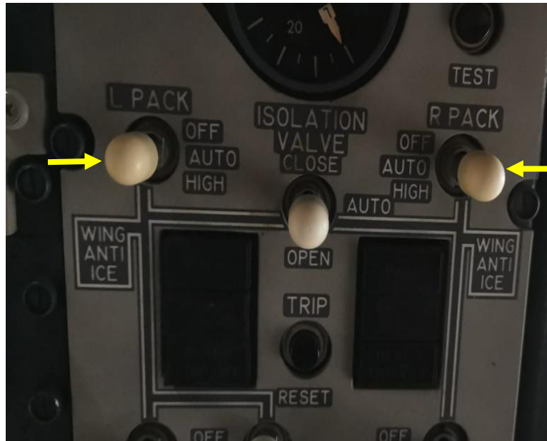
Figure 5: The aircraft pneumatic panel showing the pre-flight set position of the air-condition packs toggle switches (Bleed 1 & 2) on Auto.
